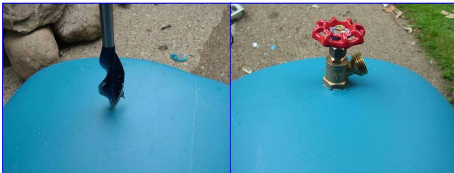
2. Drill a 1" hole near the bottom. Place some adhesive/sealant around the threads of the boiler drain and screw in. Be sure to have the opening to the side to leave plenty of room for hose.
